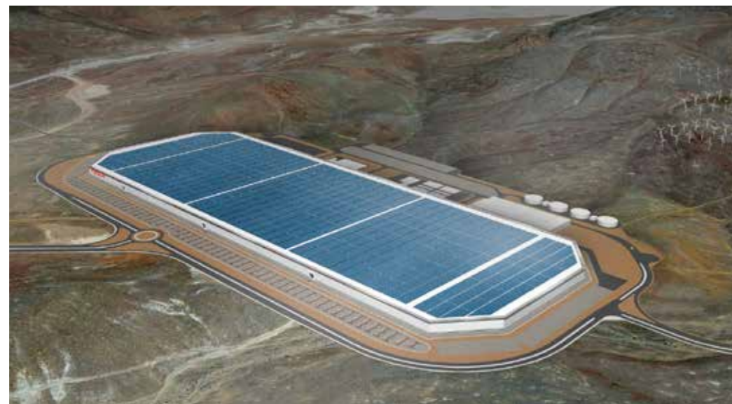
That's how it will look like when it will be completed: Tesla's Gigafactory will produce up to 500,000 rechargeable batteries per annum.
